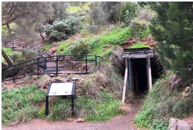
The portal to the lower adit at Wheal Watkins
